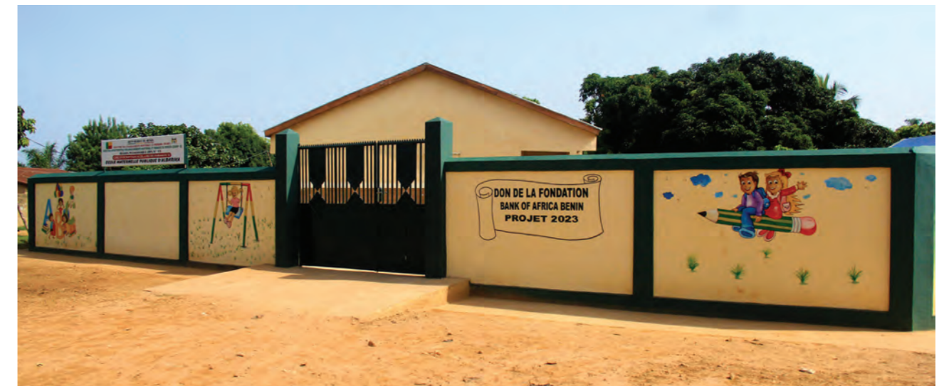
Renovation of Albarika nursery school in Parakou
