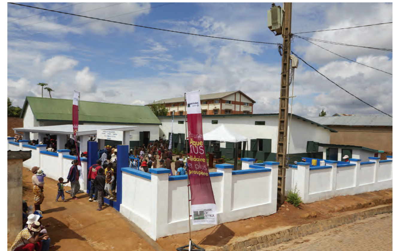
Renovation of a primary school
